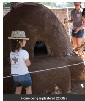
Horno being re-plastered (2000s)
